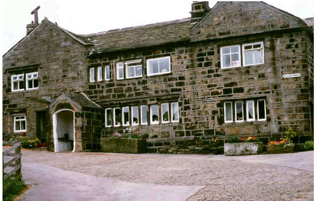
Figure 16: Ellistones Farmhouse, Elland. Elland Flags and sandstone slate roof.
