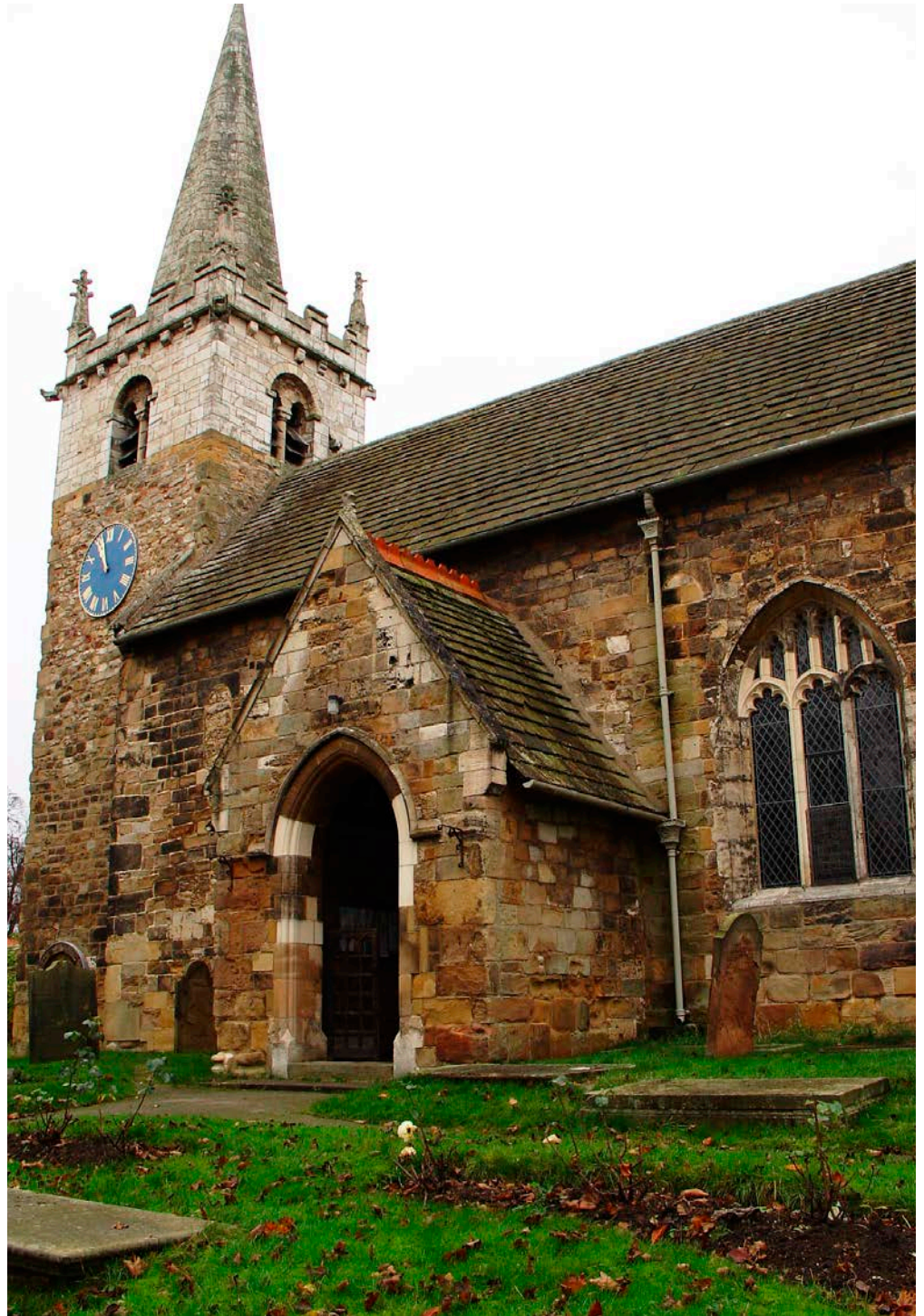
Figure 25: All Saints Church, Ledsham. Thornhill Rock Sandstone and Dolomitic Limestone.
