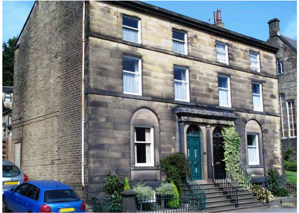
Figure 13: Houses, Holmfirth. Huddersfield White Rock.
